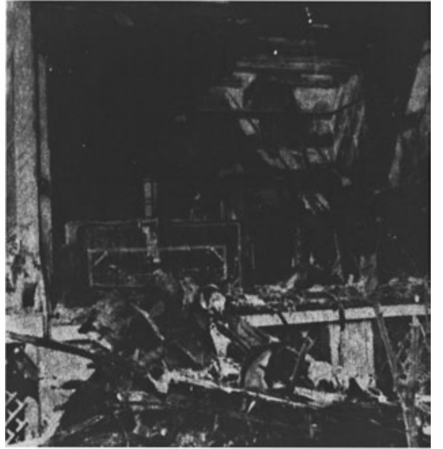
BURNED HOME ON SOUTH WARREN STREET
