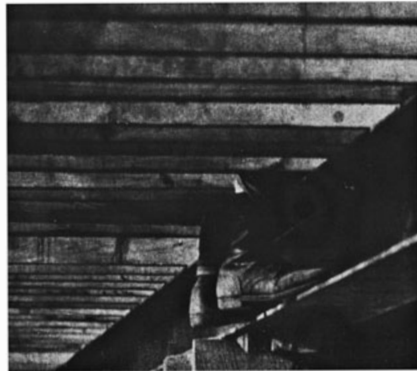
PHOTO EDITOR JAMES H. PEPPER WAS LET LOOSE AT THE CONSTRUCTION SITE OF THE INTERSTATE HIGHWAY THROUGH MONTGOMERY, AND THIS IS WHAT HE FOUND UNDER A NEW BRIDGE.
