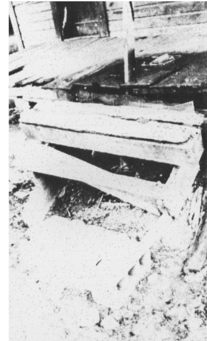
CRUMBLING FRONT PORCH
