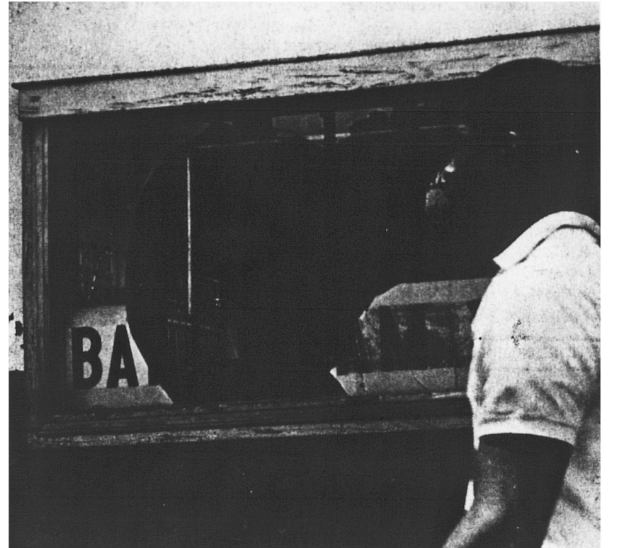
DAMAGE IN BIRMINGHAM
